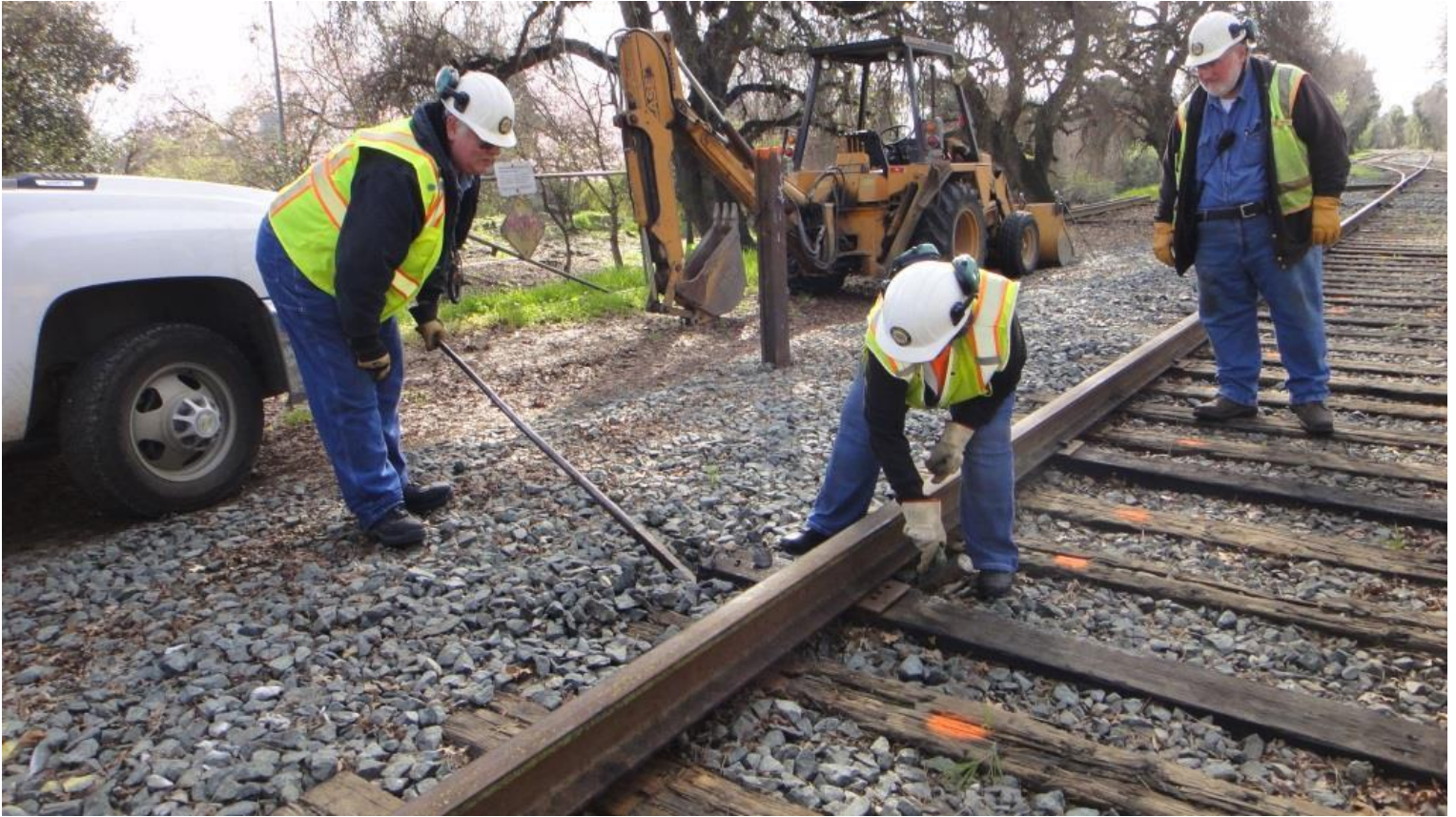
Chris nips-up the tie as Pam sets spikes
