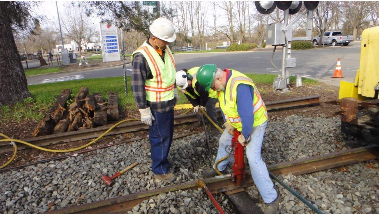
Then, Tom drive the set spikes the rest of the way in with the pneumatic spike-driver
