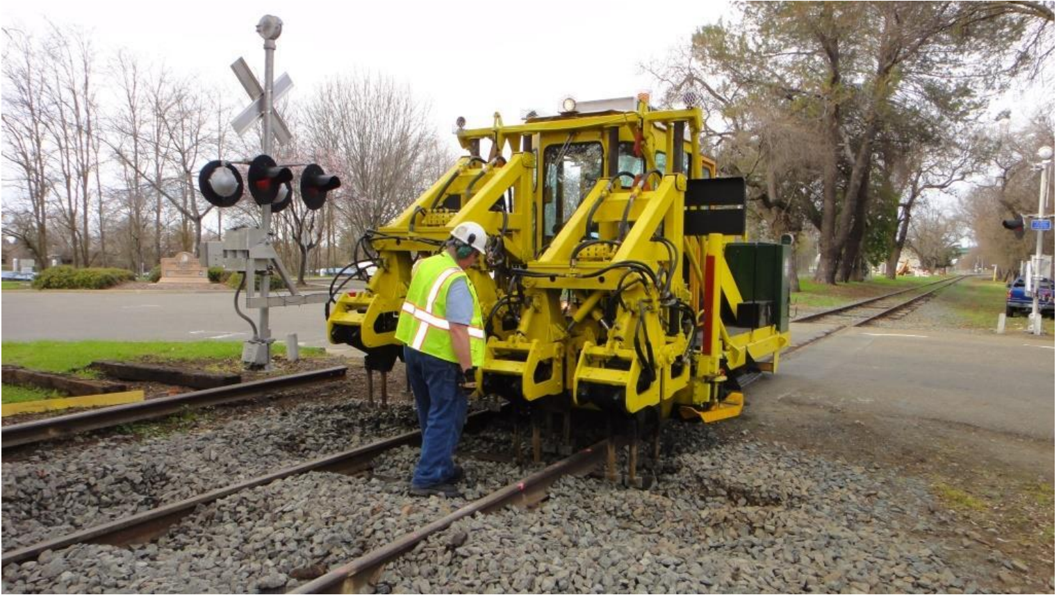
Meanwhile, Steve in the tamper guided by Chris begins tamping the new track
