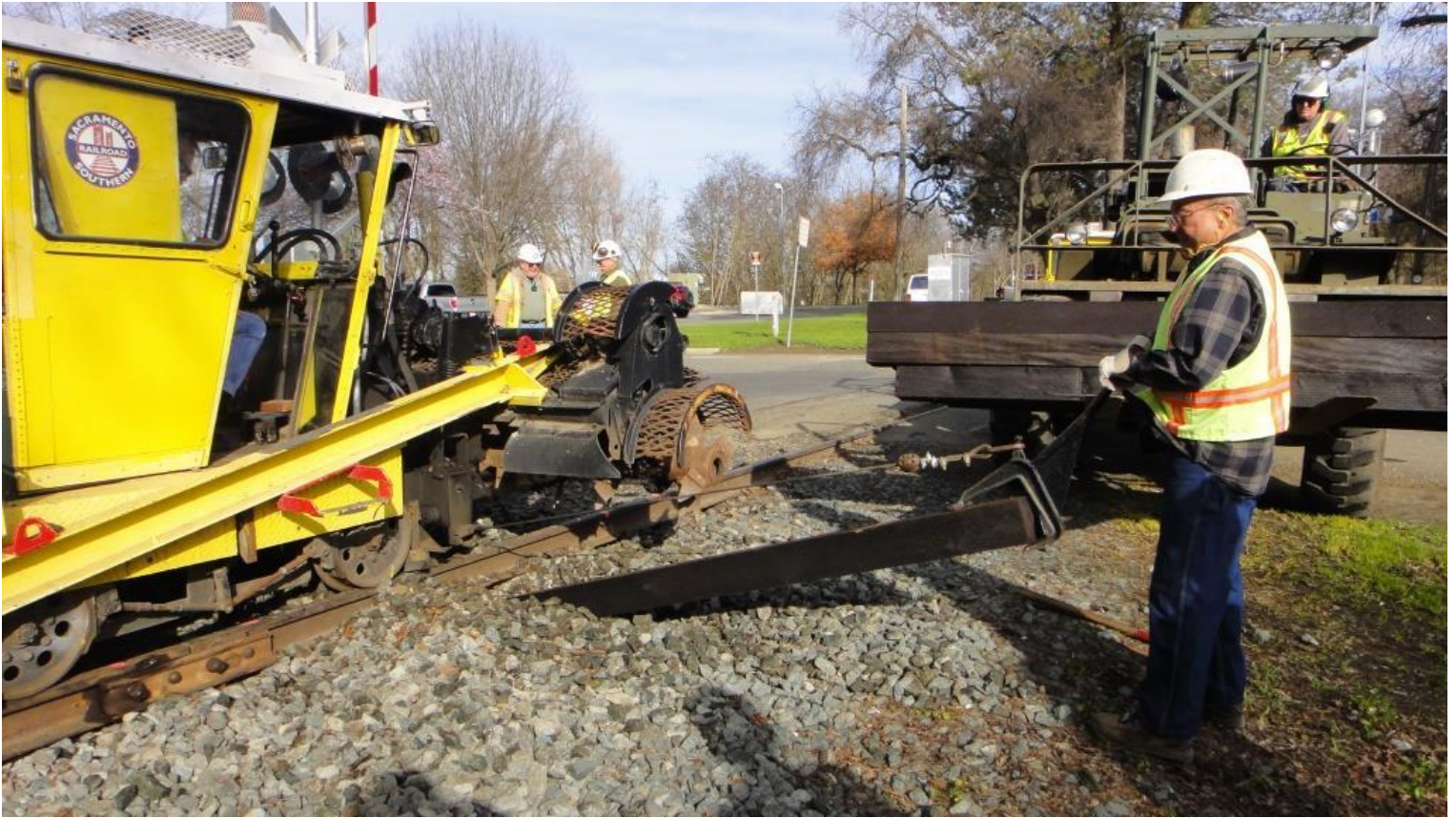
Oops! That's a little steep – with Alan in the scarifier, John guides a new tie under the north end
