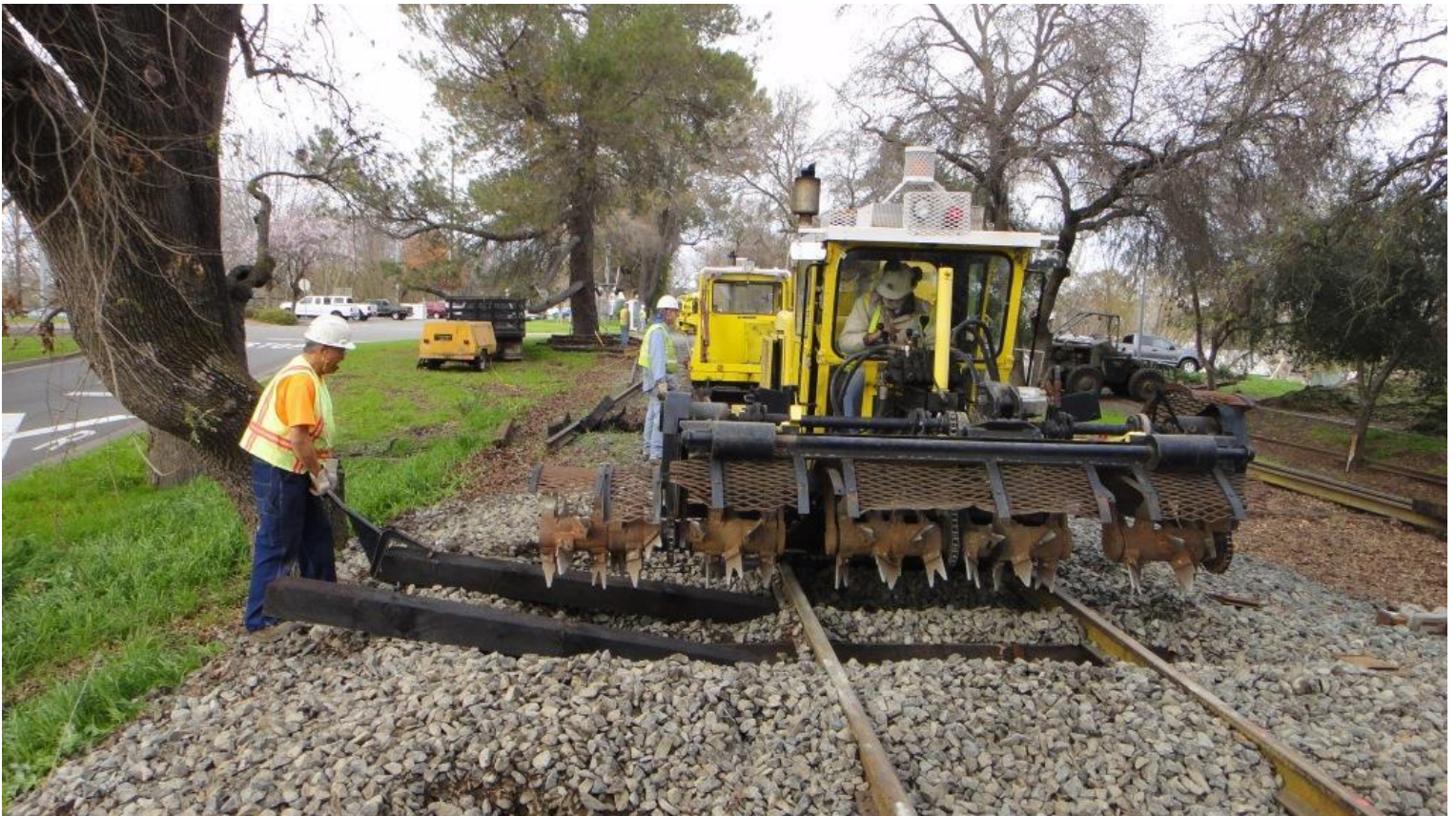
At the south end, John and Alan work to pull in more ties
