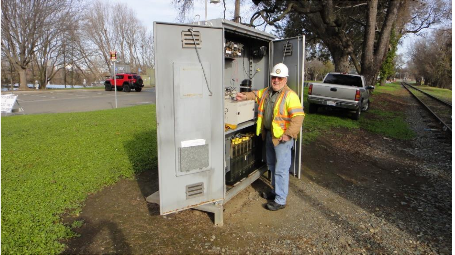
Signals Joe kept us safe by deploying the crossing gates at Front Street when we needed to cross
