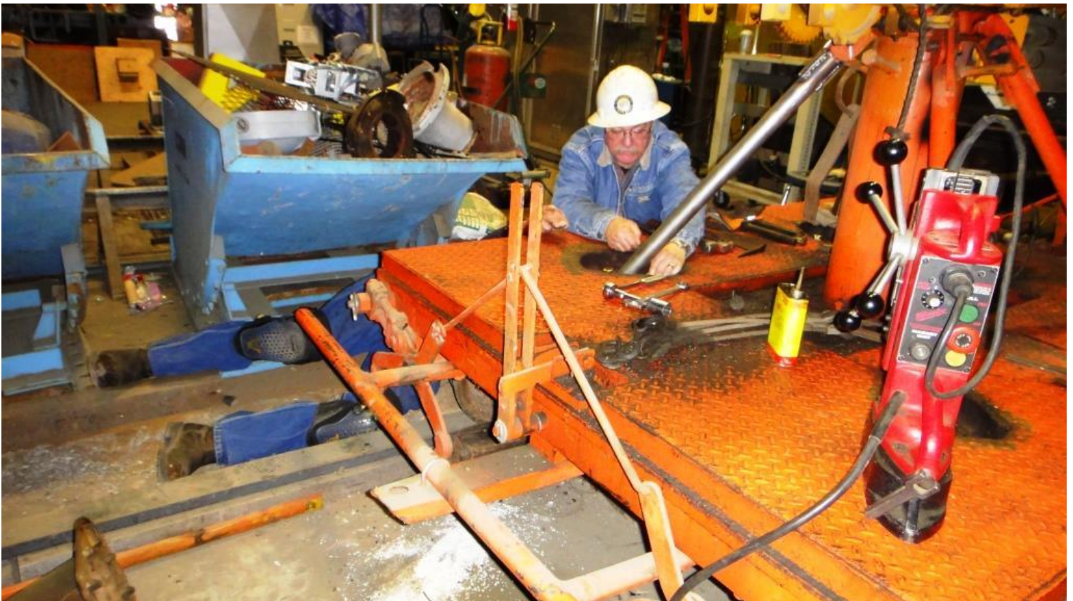
Mike H. and Cliff (on the floor) bolt the new support-bracket onto the tie-crane
