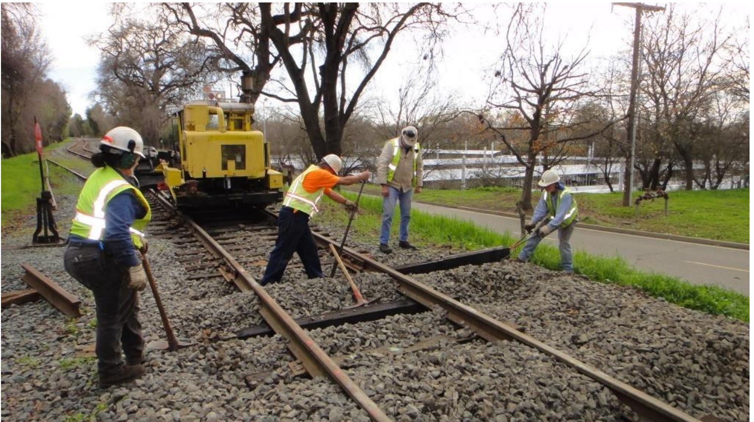
The new tie just wouldn't go in so Heather, John, Alan, and Mike M. struggle to remove it before trying again
