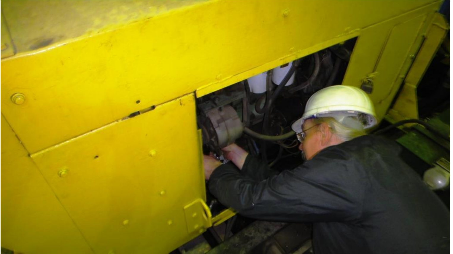
Fred installs the new air-dryer/oil-separator on the tie-shear
