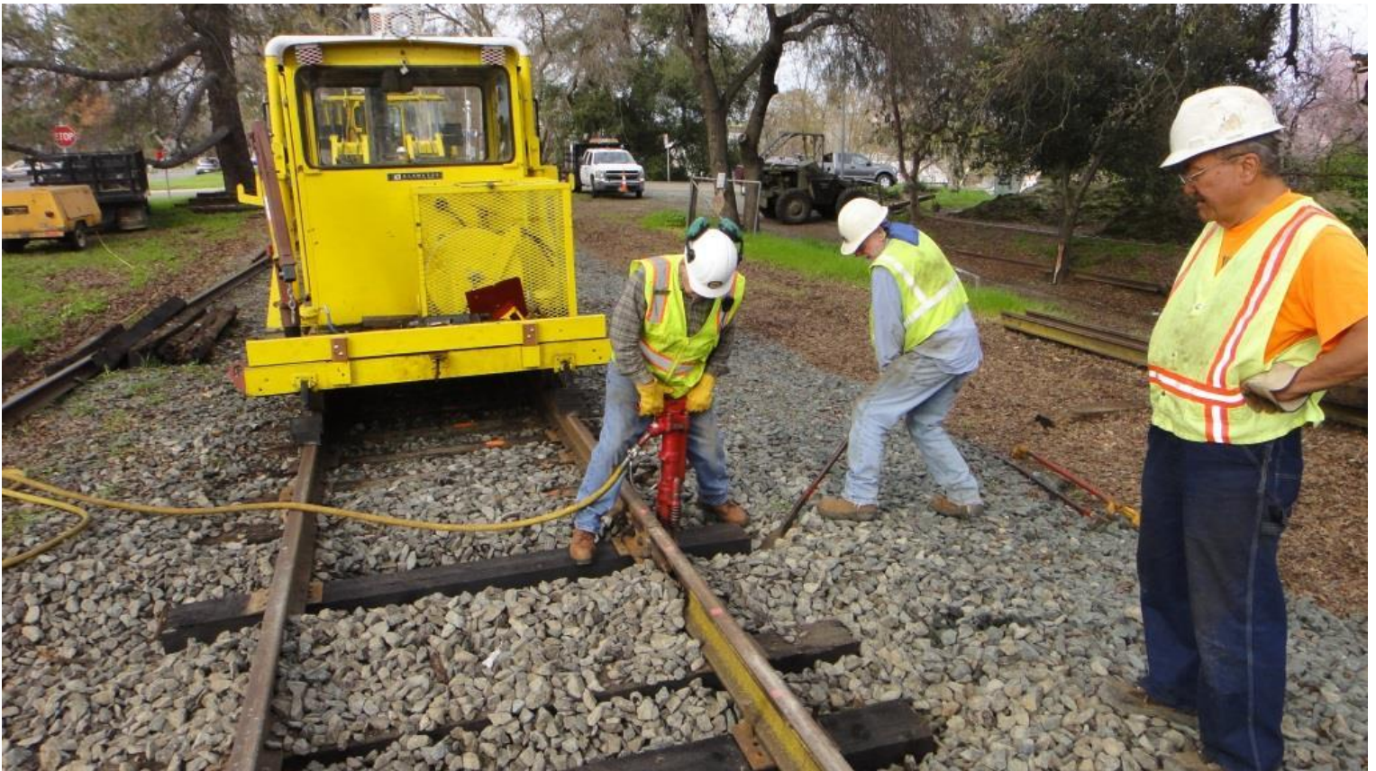
With the last ties finally in place, Mike W. spikes while Mike M. nips. John keeps an eye on 'em...
